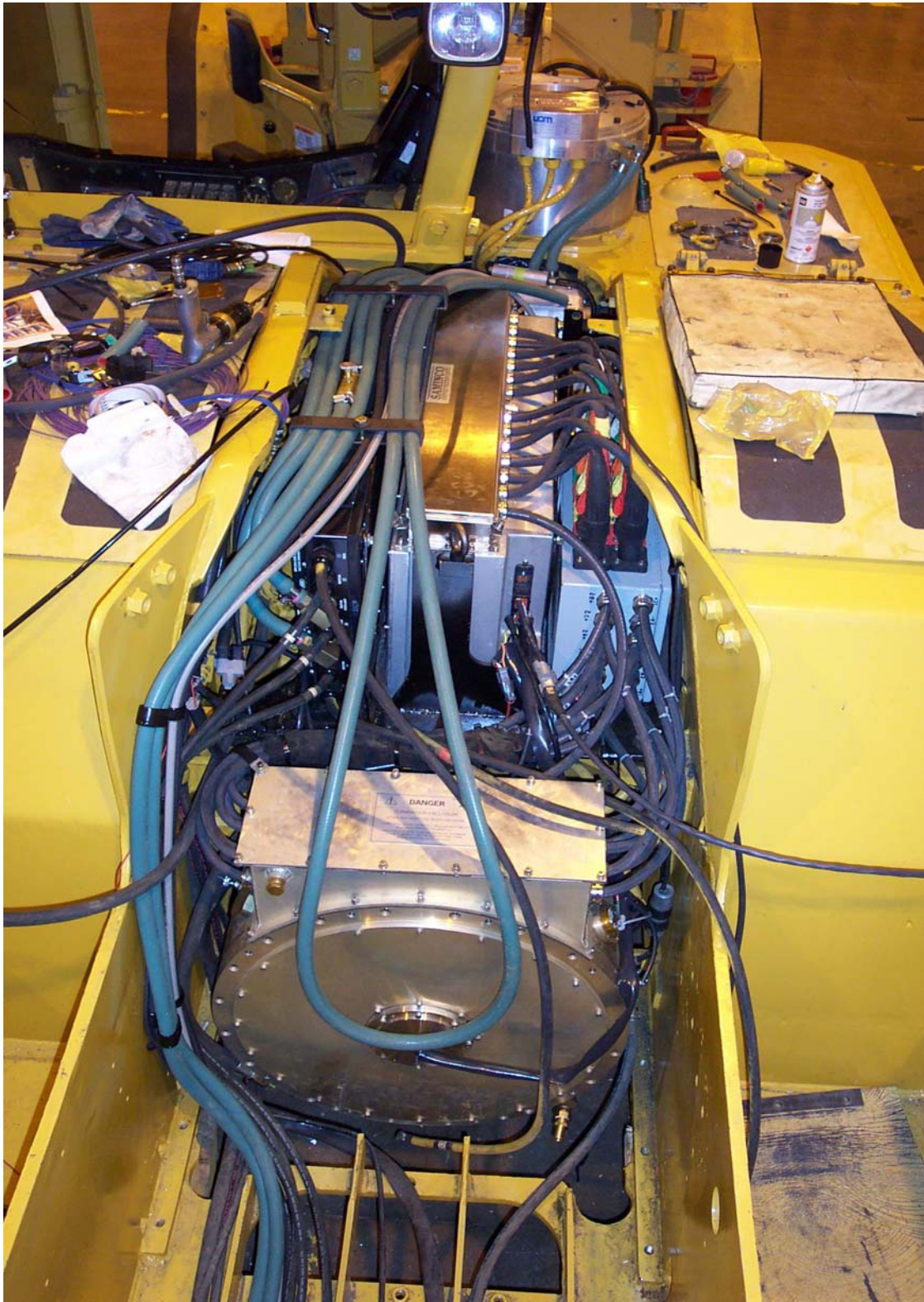
Figure 22: DRS PA44 motor, Saminco motor controller and motor contactor box
